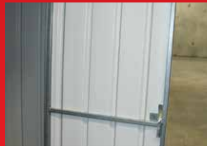
Upgrade to Steel Frame Door and Opening
